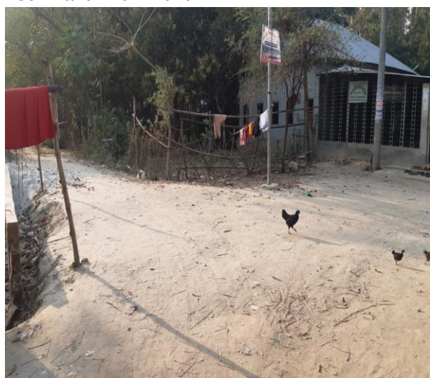
WARD-6 and 7 : (R1) Construction of RCC road and Drain at nowani Azahar-Afser Road to Pipulia Babur Ali House Via Harez Rice Mill. R-01= CH: 785 m and D-01 = 670 m.
