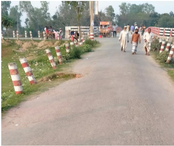
WARD-1 and 2: (R10) Construction of road and Chanchhania bera- Madhupur Road to Ichhamai R10-CH-1465 m. And D02: CH: 434
