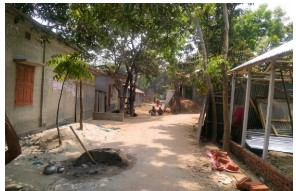
SP-R-023 Rehabilitation of BC road at Chanchania Mozid Haji house to Teghore more
