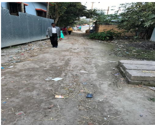
WARD-6 and 7 : (R1) Construction of RCC road and Drain at nowani Azahar-Afser Road to Pipulia Babur Ali House Via Harez Rice Mill. R-01= CH: 785 m and D-01 = 670 m.
