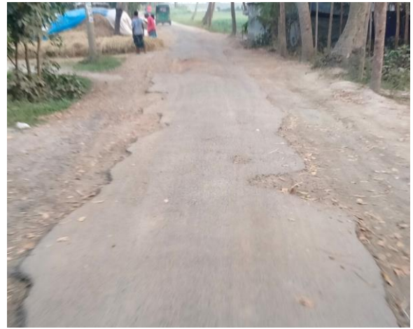
WARD-1 and 2: (R10) Construction of road and Chanchhania bera- Madhupur Road to Ichhamai R10-CH-1465 m. And D02: CH: 434
