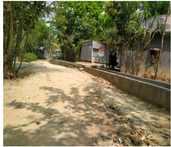
SP-R-105 Construction of RCC road at Santhia Babur Ali house to Mannan fokir house.
