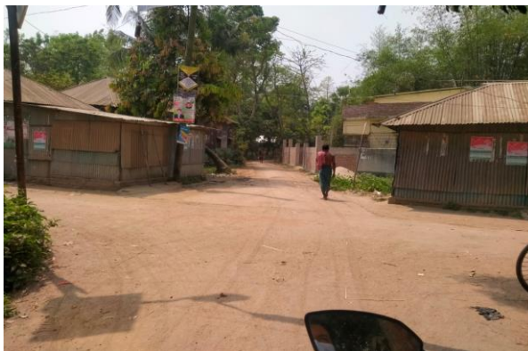
SP-R-023 Rehabilitation of BC road at Chanchania Mozid Haji house to Teghore more
