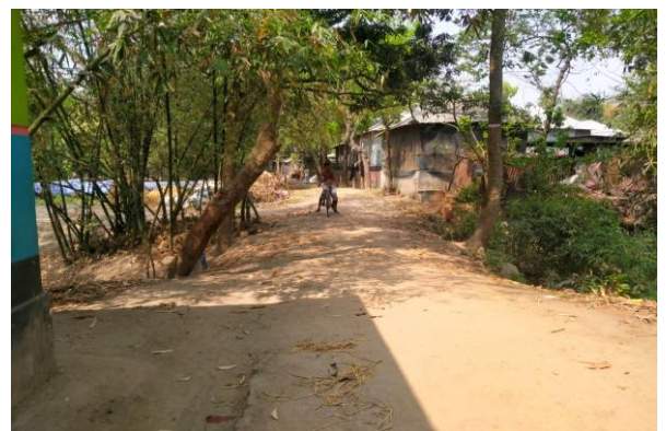
SP-R-104 Rehabilitation of RCC road at Santhia Rohim mollah house to Santhia – Chakla road Via mosque at moej house
