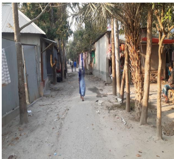
WARD-1 and 2: (R10) Construction of road and drain at Chanchhania bera- Madhupur Road to Ichhamati River R10-CH-1465 m. And D02: CH: 434
