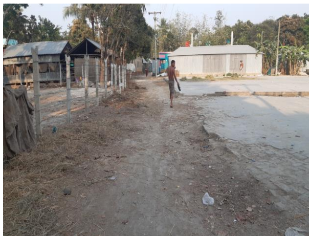
WARD-6 and 7 : (R1) Construction of RCC road and Drain at nowani Azahar-Afser Road to Pipulia Babur Ali House Via Harez Rice Mill. R-01= CH: 785 m and D-01 = 670 m.
