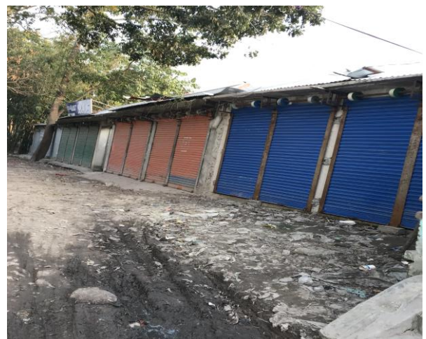
WARD-5 (D-3) CONSTRUCTION OF RCC DRAIN AT BASED SHOP TO NIZAM CHAIRMAN HOUSE VIA AZHER HOUSE. LENGTH- 305
